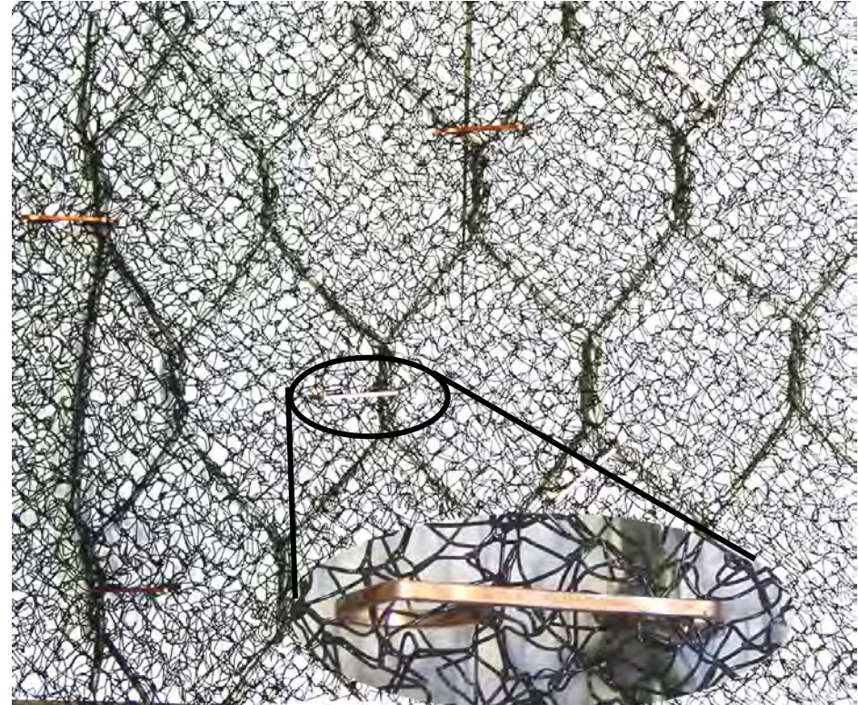
Fixing of a steel meshwork on a steel wire with staples
